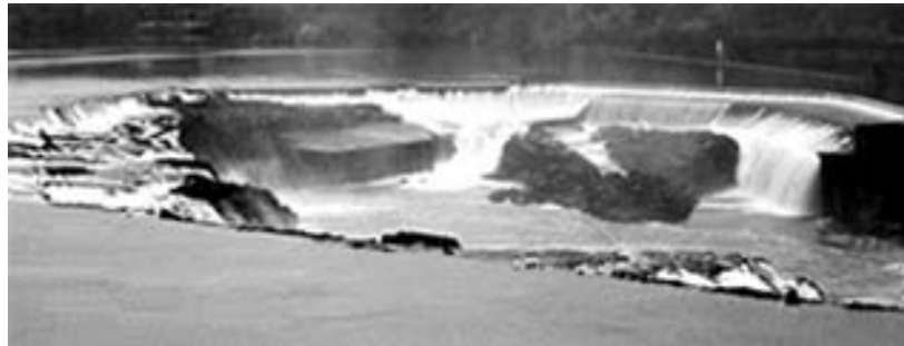
Willamette Falls; Sullivan Hydroelectric Facility.
